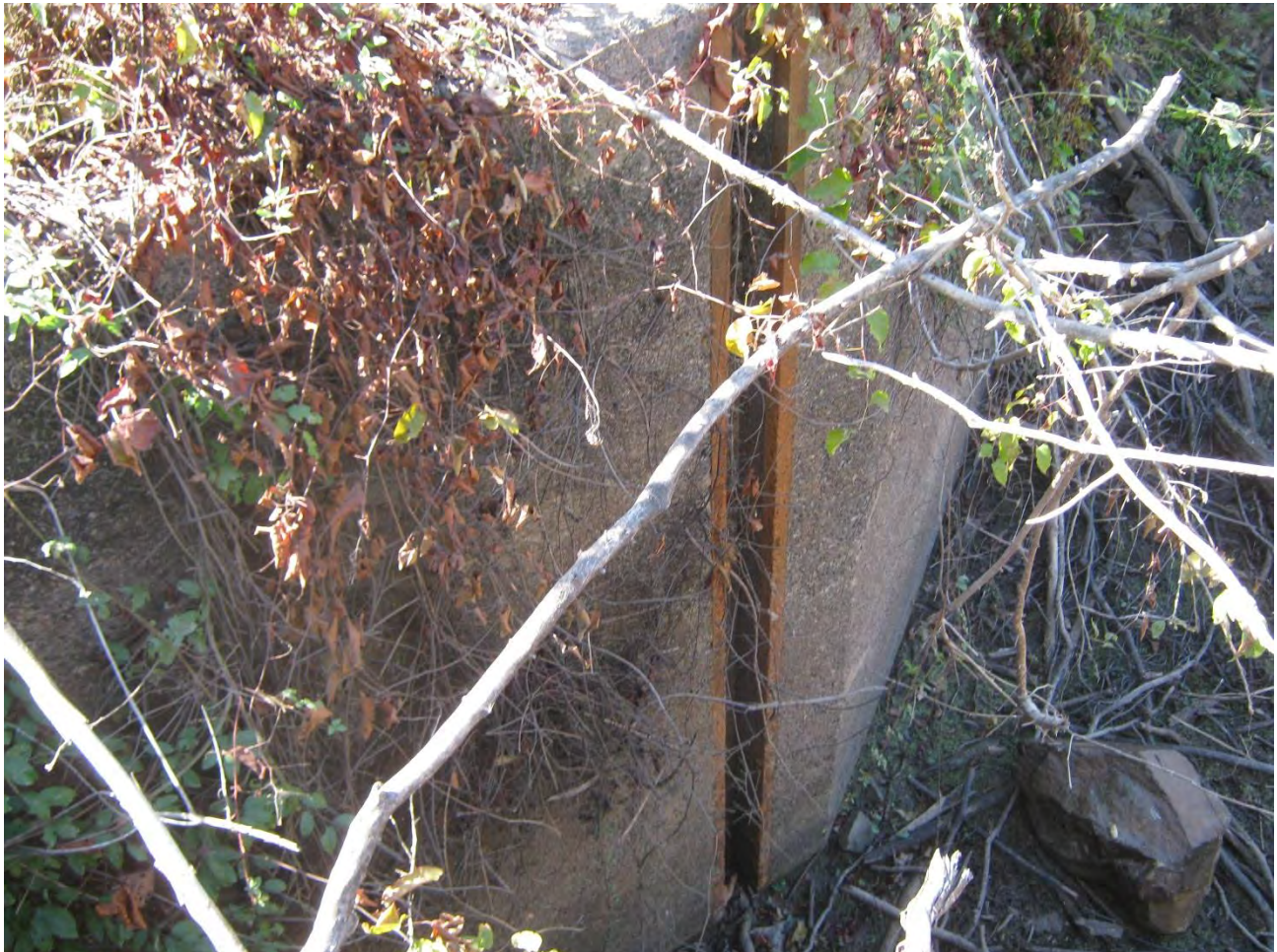
Figure 6 - Area 1, Debris and guide frame. South side of the southern 60" concrete pipes inlet.
