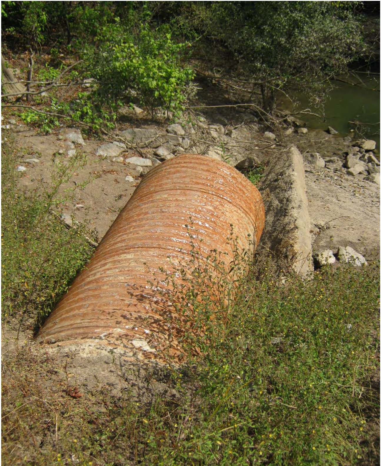
Figure 9 - Area 4, Outlet end of 36" CMP replaced by the USFWS.
