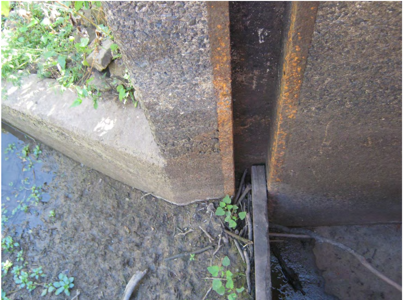
Figure 8 - Existing 36" CMP inlet 5440 feet east of Area 1. Typical guide installation. Note sediment on upstream side.
