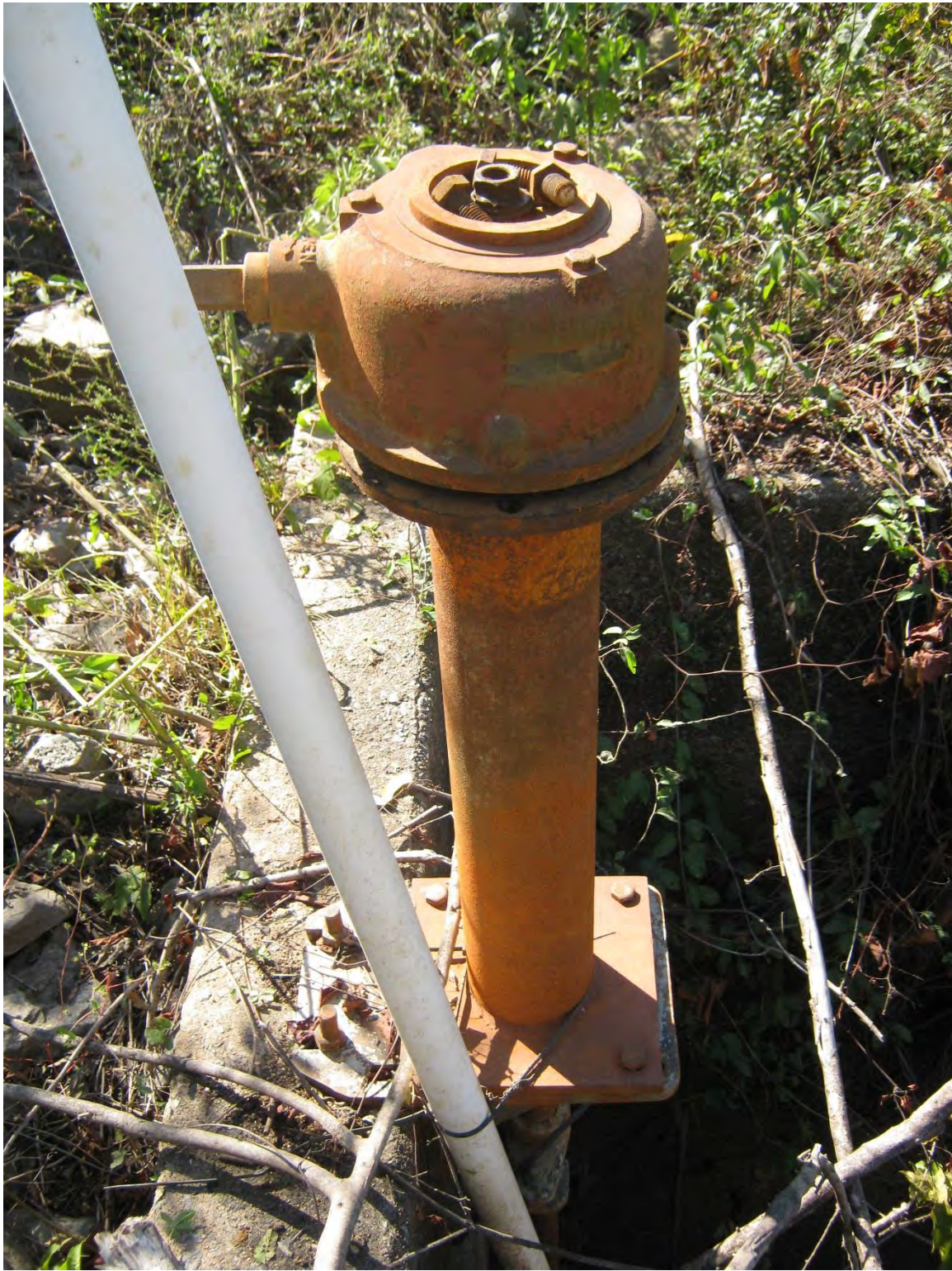
Figure 3 - Area 1, Existing Gate Mechanism (Note that it has been disassembled.)
