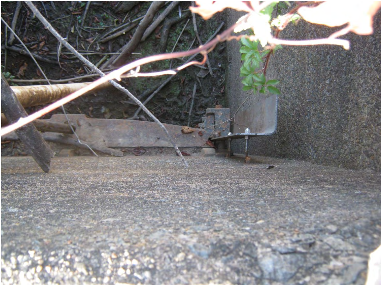
Figure 4 - Area 1 - Existing southern slide gate. Note that the anchor bolts are not connected.
