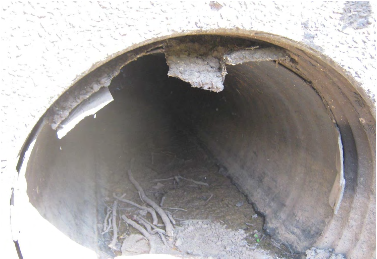
Figure 7 - Existing 36" CMP, 5440 feet east of Area 1. Typical liner installation. Note the poor liner adhesion at the pipes entrance.
