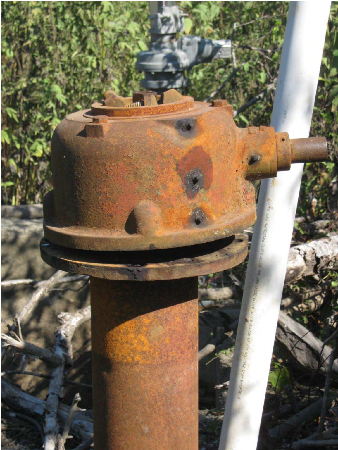
Figure 2 - Area 1, Existing Gate Mechanism (Note that it has been disassembled.)
