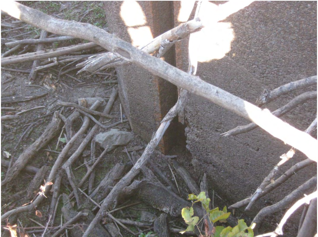
Figure 5 - Area 1, Debris and missing guide frame and concrete spalling. North side of the southern 60" concrete pipes inlet.
